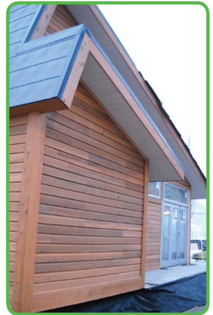
The West House demonstration laneway house is on display at the LiveCity Yaletown site, right next to Vancouver House.
